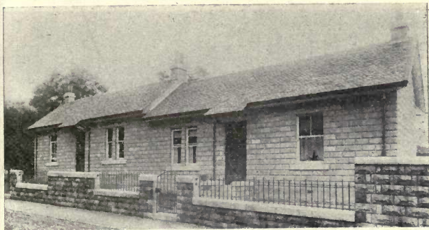
FIG. 5—TWO-FAMILY CONCRETE BLOCK COTTAGE AT DUNBARTON, SCOTLAND.
